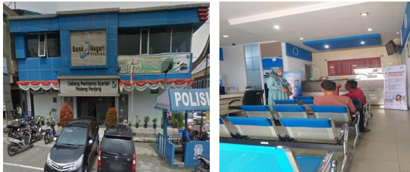
Figure 1. Condition of Facilities at Bank Nagari Syariah Sub Branch
